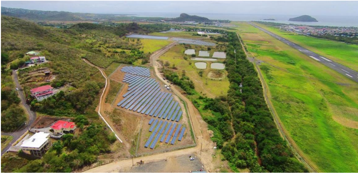
Figure 5: La Tourney Solar Plant, Saint Lucia. Source: LUCELEC
