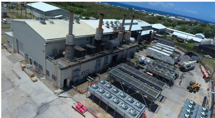
Figure 4: Needsmust Power Station, Saint Kitts. Source: SKELEC
